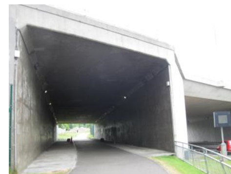
Looking towards the site through the existing underpass
